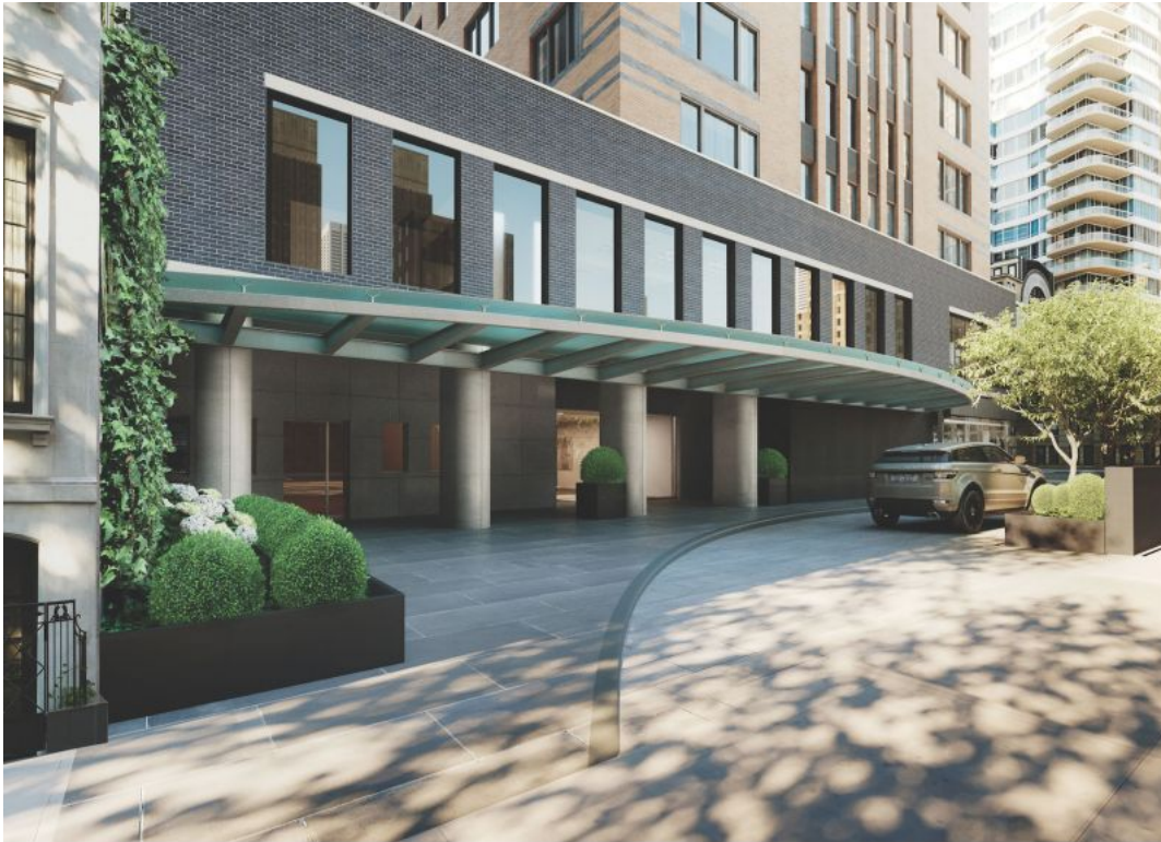
Newly Landscaped Porte-Cochere, 200 East 62nd Street.
